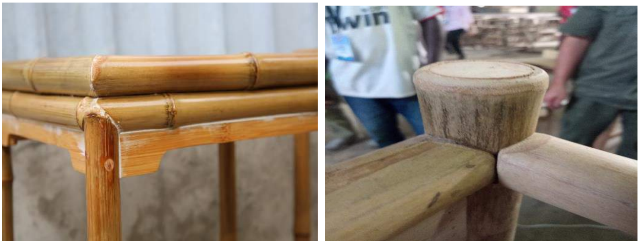
Fig 34. The two pictures above shows, joined bamboo culms with the aid of white glue and pins
